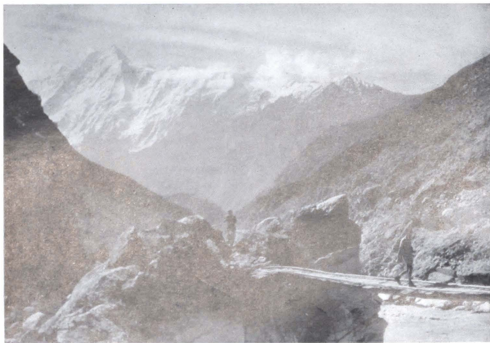
18a. Bridge near hot spring above Chalt—Rakaposhi in background
