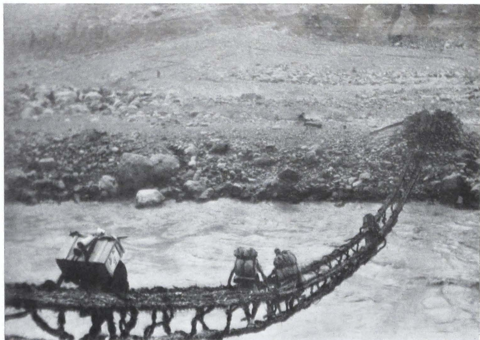
7b. Rope bridge near Matun Das
